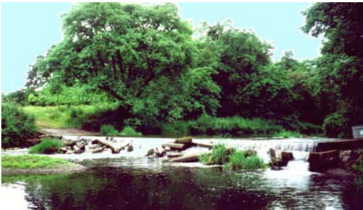
Photo 1-2: Lower Rickreall Creek at Villwoks Dam, a concrete ford over the stream at River Mile 7.5. The lower section of the Rickreall is characterized by a channel of low gradient that is somewhat entrenched. The riparian zones are narrow but well developed with mature hardwoods. Land-use along this section is agriculture beyond the riparian zone.
